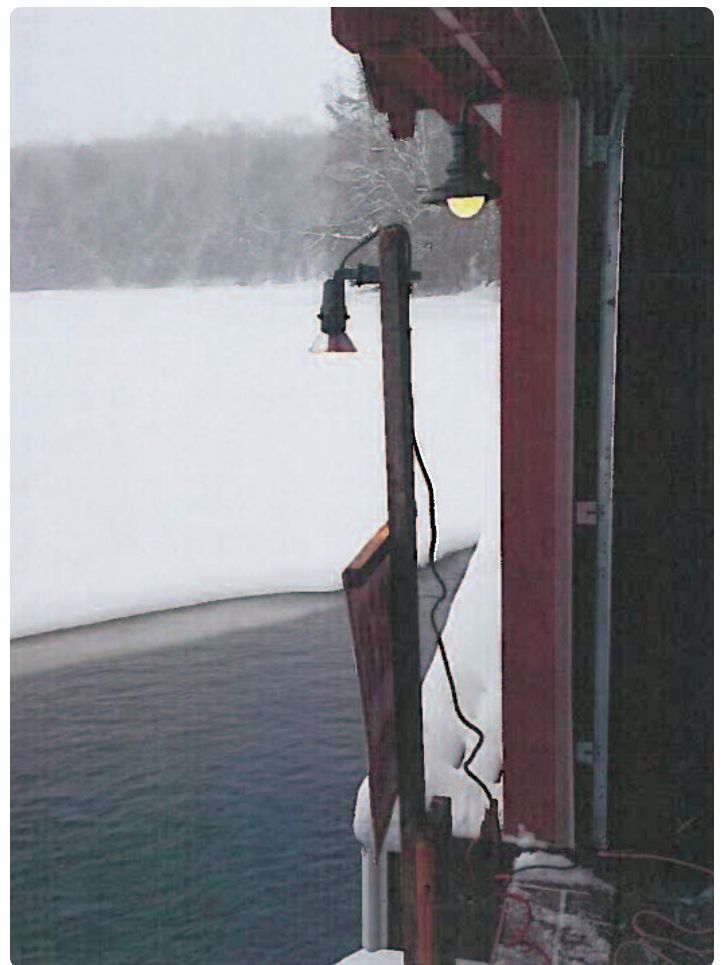
The light is angled down to illuminate the warning sign.
